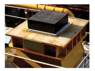
As the bearings are designed to be flexible they greatly reduce the transmission of vibration from any external disturbance.
